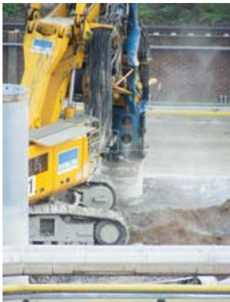
Drilling the hole for the pile foundation
