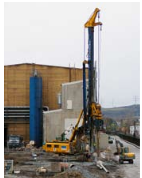
Rotary boring machine in action
