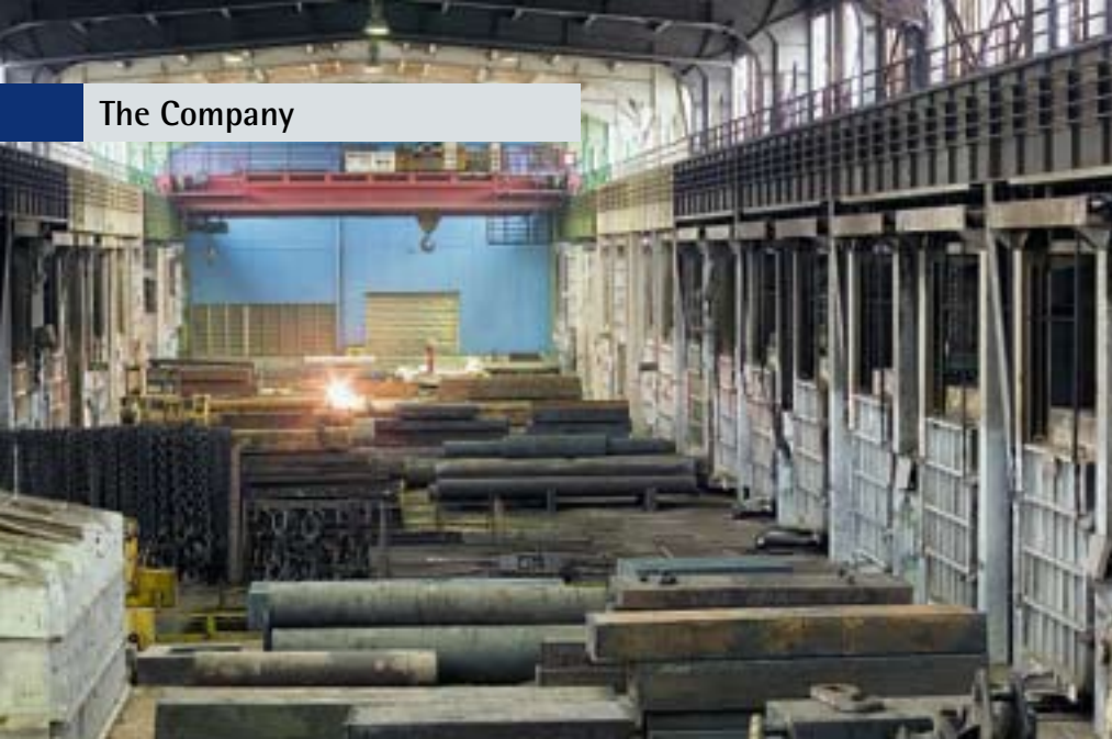
Overall view of the annealing shop
