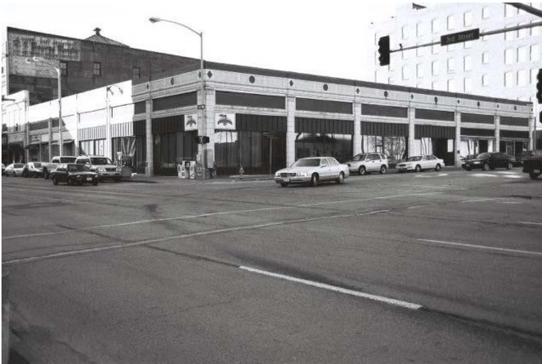
View of the south and east elevations, looking northwest across the intersection of Main and Third Streets.
