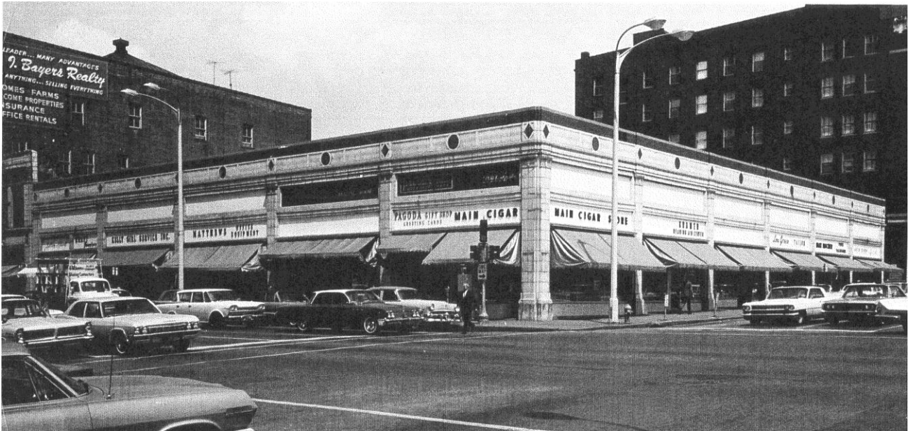
This historic image documents the building at 202 W. 3rd Street in c.1965. When compared to the previous, 1926 image, it appears that a parapet with a decorative balustrade has been removed from the building's roofline.
