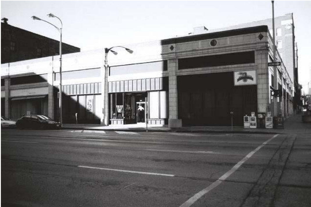
View of south elevation, looking north across West Third Street.
