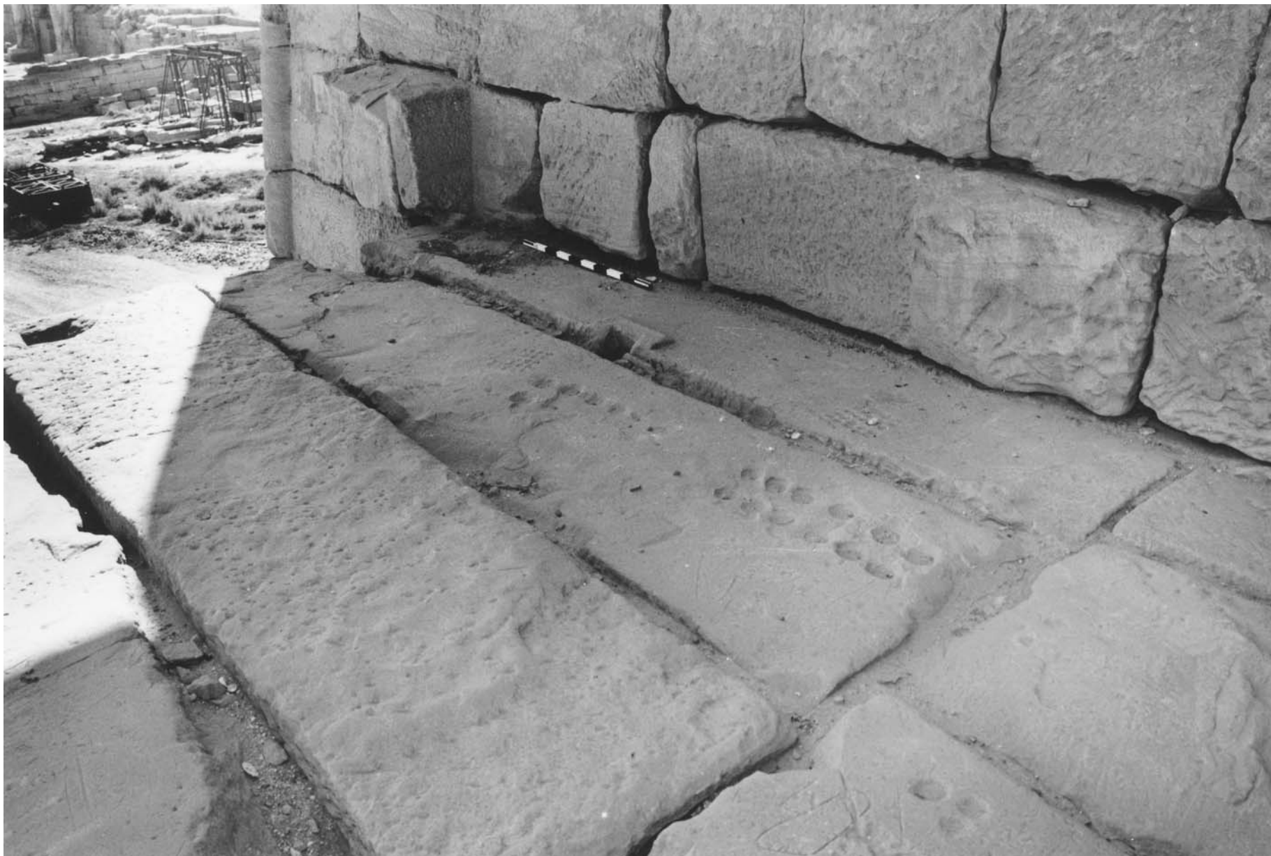
Figure 3. Remains of the Cornice and Balustrade Blocks at the Southeast End of Row A above Block A1 Where They Are Still Anchored in the Face of the Pylon
