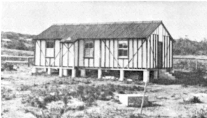
This is the old hostel. It was used to house outpatients coming from the country to attend Sydney hospitals.
