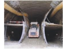
Fig. 10: core method Uetliberg
