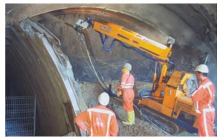
Fig. 38: sprayed concrete test for controlling rebound
