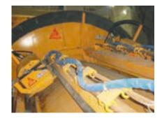
Fig. 46: Round arch spraying robot on the tunnel boring machine of the JV TAT, Gotthard base tunnel, section Bodio
