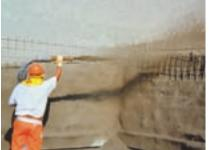
Fig. 26: nozzle man spraying manually
