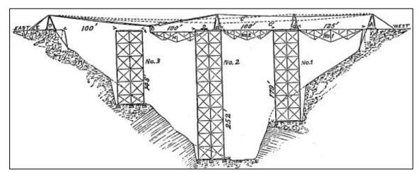
Figure 4. Erection of Piers 2 and 3 and Spans 2, 3, and 4.
