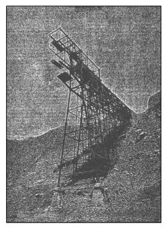
Figure 11. View showing newly built west pier and use of traveler to build out cantilever span.
