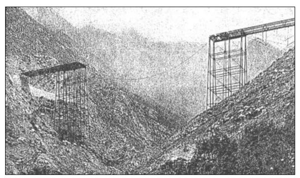
Figure 7. Unsupported rail spanning between Piers 1 and 3 after the accident.
