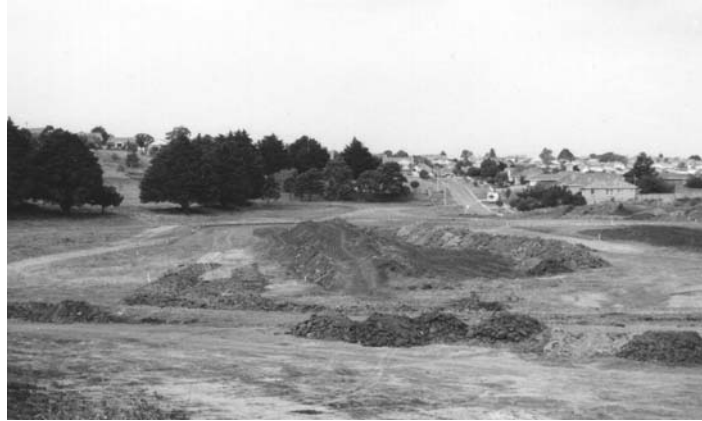
Aberfeldie Track under construction 1971
