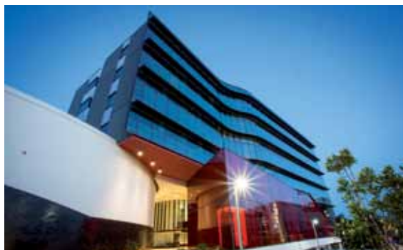
The new Griffith Business School building at the Gold Coast campus.
