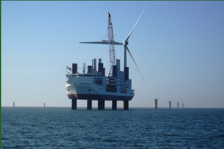
The Resolution on site during offshore wind turbine installation at the Lynn Offshore Wind Farm
