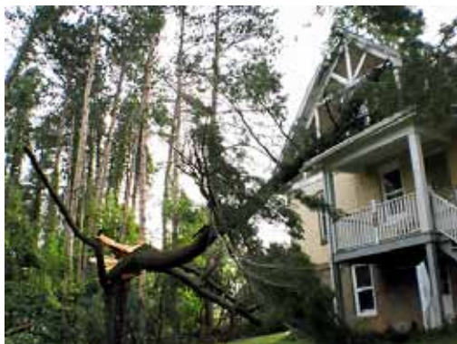
Summer storm damage to the Hutton House
