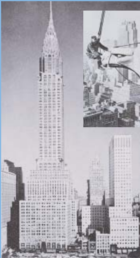
Courtesy of the American Iron and Steel Institute
