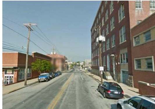
Like James street, Lemon Street contains between 8 and 10 feet of excess pavement.
