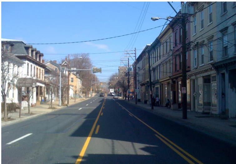
In Bethlehem, PA, an unnecessary and overlong turn-lane has eliminated a block of curb parking severely impacting adjacent businesses.
