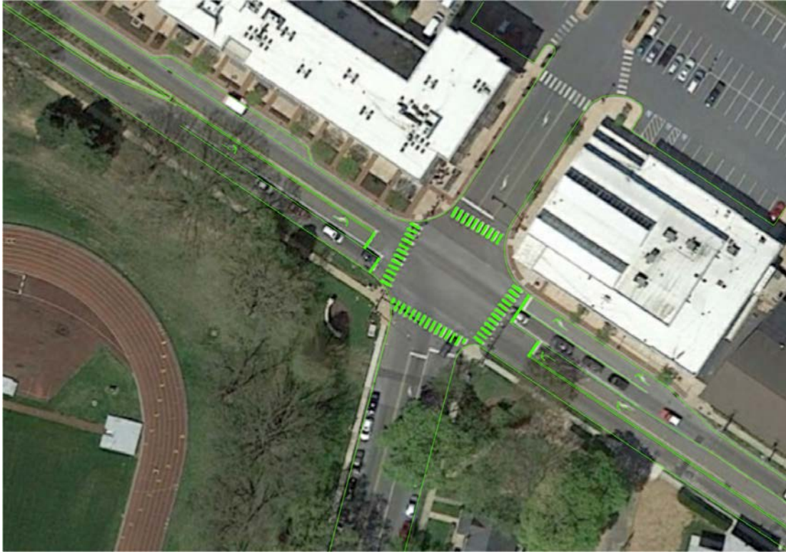
Central segment of Harrisburg Pike: Existing Conditions
