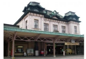
7 Heritage related to transport and trade of coal produced from Chikuhō Coalfield
