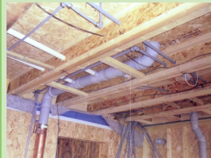
Figure 17: Integral garage ceiling during second fix
