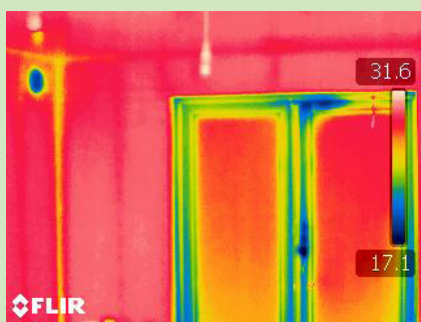
Figure 11: Living room dynamic insulation supply louvre in external wall and heat loss around French doors
