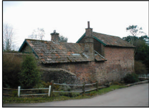
Left: Selworthy Farm with the former farmhouse in the background, 17th-19th century farm buildings on the left, and the remains of an orchard on the hillside beyond. Right: former outbuildings, converted to residential use, probably in the late 19th century. The Bridgwater pantiles may have replaced thatch.
