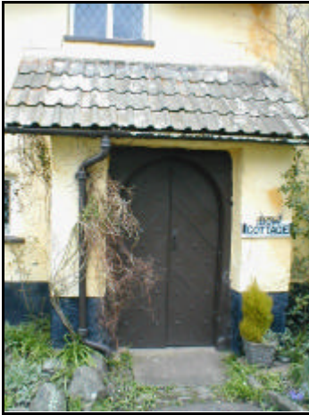
Cottage detail at Selworthy Green. Left: double-doors of opposed diagonal plank construction within a Gothic-arched frame. Centre: steps up to Clematis Cottage. This dates from the early 19th century and is in “cottage ornee style” which often included use of thatch. Right: entrance detail at Clematis Cottage, showing a vertical plank door with ribbed panels and edges. The variety of detail, here with ogee-headed openings, and diamond paned leaded-
