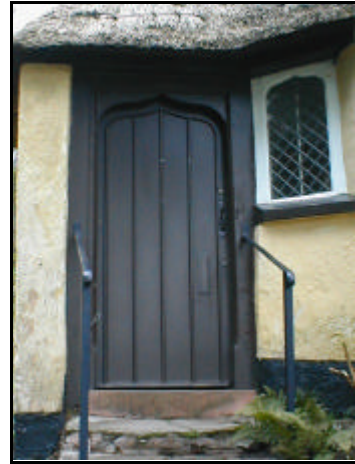
Cottage detail at Selworthy Green. Left: double-doors of opposed diagonal plank construction within a Gothic-arched frame. Centre: steps up to Clematis Cottage. This dates from the early 19th century and is in “cottage ornee style” which often included use of thatch. Right: entrance detail at Clematis Cottage, showing a vertical plank door with ribbed panels and edges. The variety of detail, here with ogee-headed openings, and diamond paned leaded-
