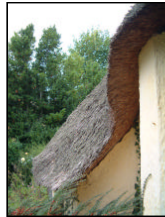
Thatch and lime-washed render at Selworthy Green
