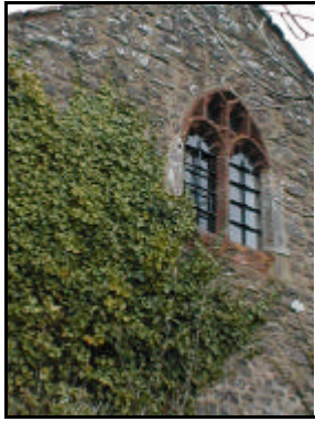
Listed Buildings in Selworthy. Left: Gable end of the Tithe Barn with cinquefoil headed two-light window, probably late medieval. Centre: Lorna Doone, Selworthy Green has late medieval origins with evidence of smoke-blackening to roof timbers Right: rear of Periwinkle Cottage with projecting lateral stack. It is possible that before the formation of Selworthy Green, this was the front elevation.
