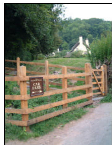
Newly installed gate and fence at the entrance to Selworthy Green.
