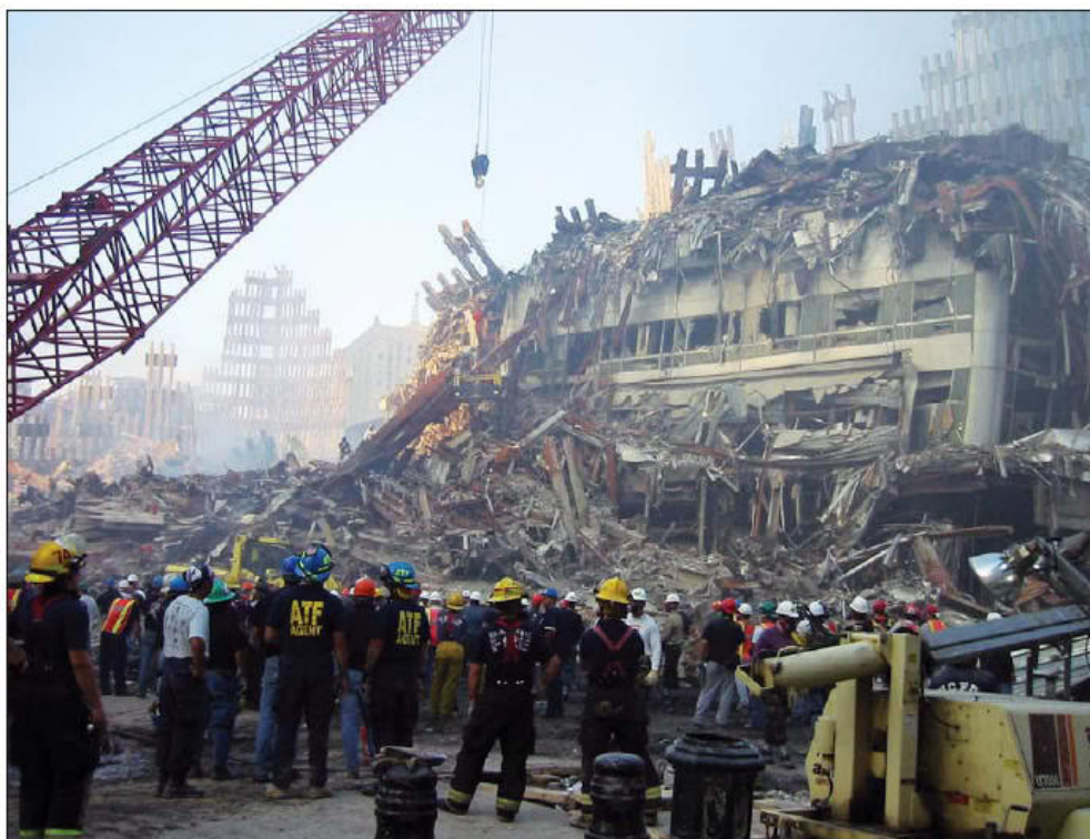
Figure 3-8 Remains of WTC 3 after collapse of WTC 1 and WTC 2.
