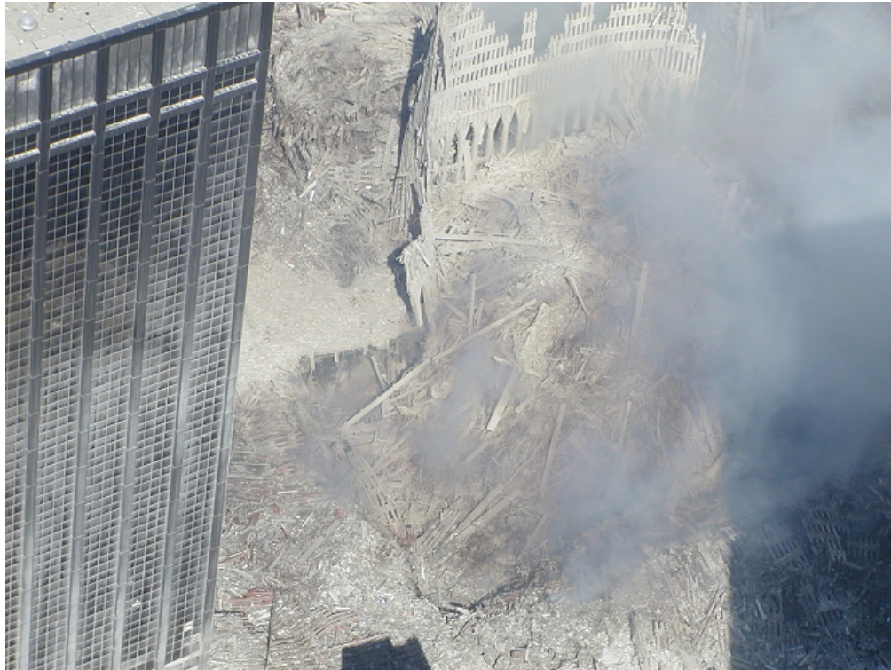
Liberty Street and WTC 2. Photo taken Sept. 13. Source: NYPD Aviation [ enlarge photo ]
