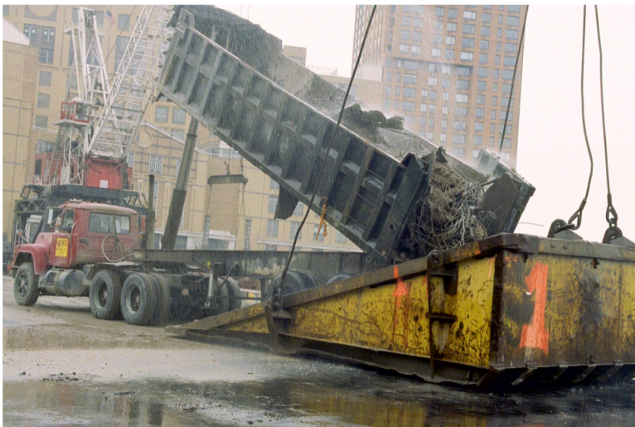
"New York, NY, March 15, 2002 -- A truck dumps debris into the bucket of a 500-ton floating crane located at FEMA's Pier 25 Loading Site, a few blocks from Ground Zero. Each day, an average of 290 loads are delivered to the pier, totaling nearly 6,332 tons. Photo by Larry Lerner/ FEMA News Photo" - the original image's metadata. See this location from an apartment above (mirror) , in Sept./Oct. 2001. 911datasets.org FOIA release 30, 42A0354 – G30D8, thanks to the International Center for 9/11 Studies.
