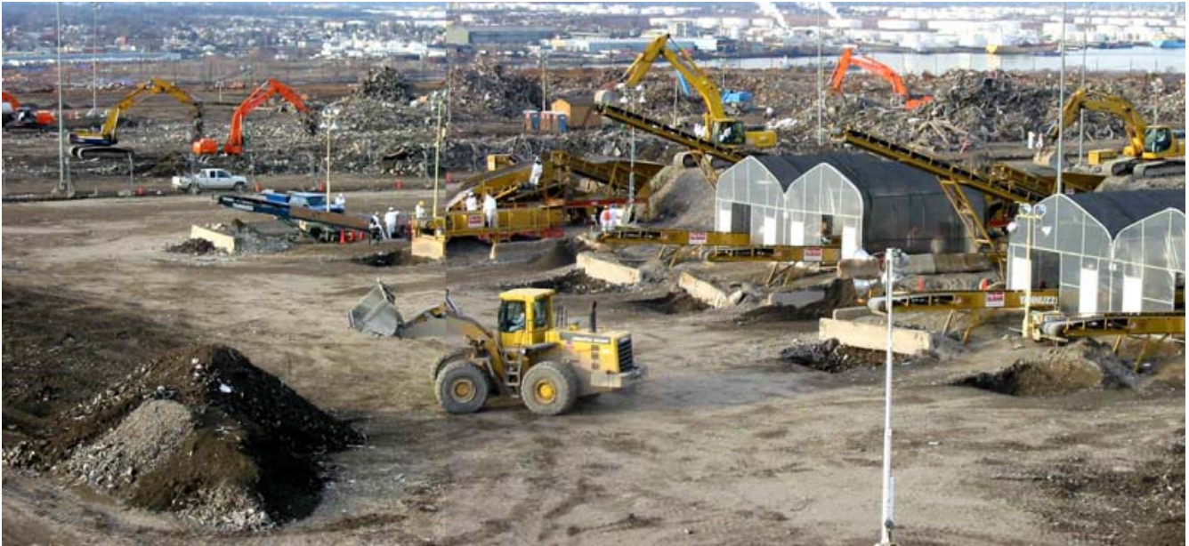
Fresh Kills processed debris from 9/11/2001-7/26/2002.(Source/date info missing.)
