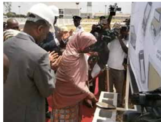
The Minister laying the foundation for the Goodluck Jonathan Multi-Purpose Hall at the University
