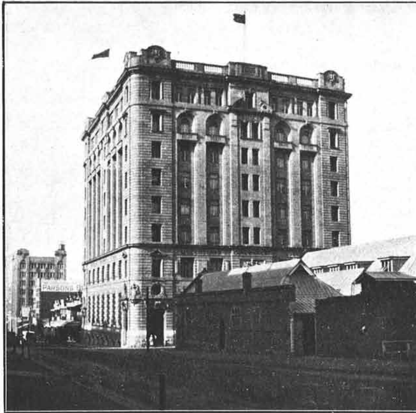
THE STATE GOVERNMENT INSURANCE BUILDING, LOOKING DOWN ELIZABETH STREET.
