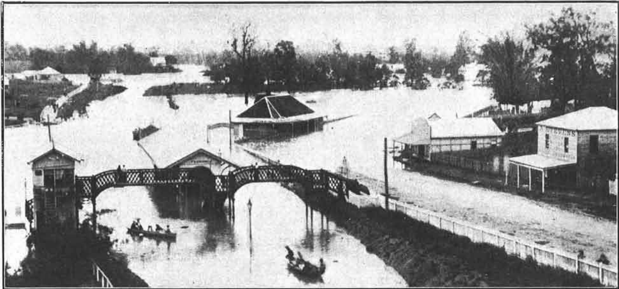
TOOWONG RAILWAY STATION UNDER FLOOD, FEBRUARY, 1893.
