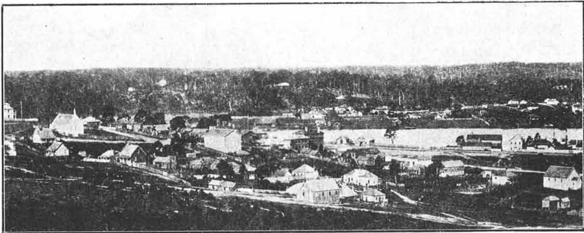
SHOWING KANGAROO POINT IN THE EARLY SIXTIES. THE WHITE TWO-STORIED BUILDING ON EXTREME RIGHT OF PICTURE WAS THE HOME OF DR. HOBBS AND USED AS THE RESIDENCE FOR SIR CHARLES BOWEN, FIRST GOVERNOR OF QUEENSLAND.
