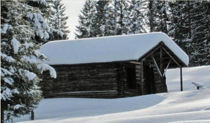
Garnet Ghost Town is filled with abandoned buildings like this one. Two of the cabins at the historic site are furnished and winterized for overnight rental.
