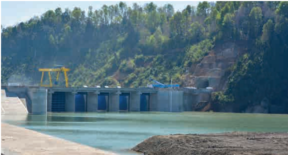
Angostura Power Plant
