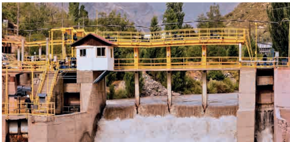
Aconcagua Power Plant
