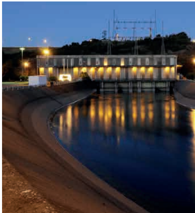
Machicura Power Plant
