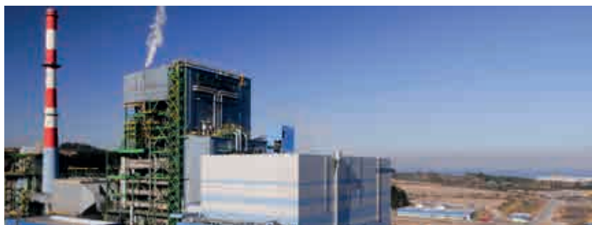
Santa María's Unit 2 Coal-Fired Thermoelectric Project, VIII Región
