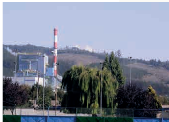
Santa María Complex's Unit 1
