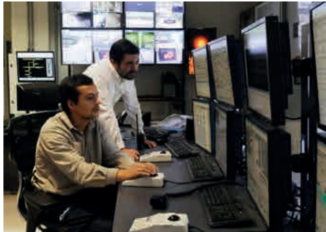
Santa María Power Plant
