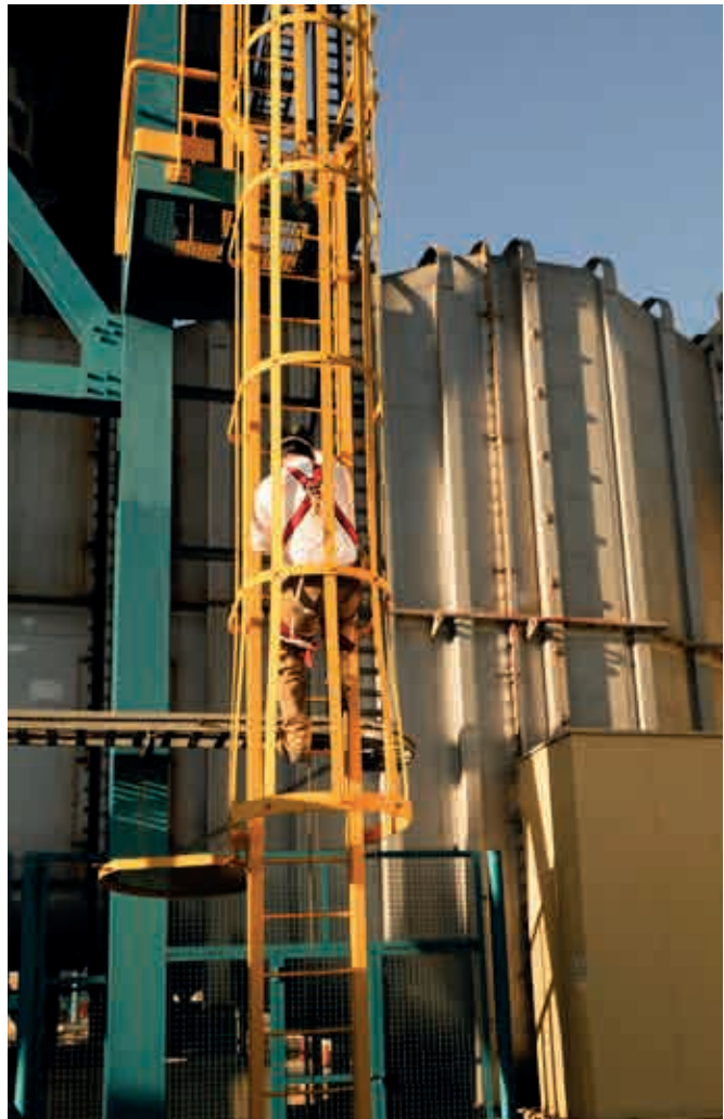
Candelaria Power Plant
