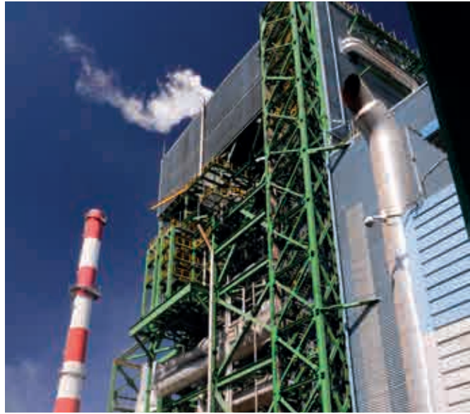
Santa María Power Plant
