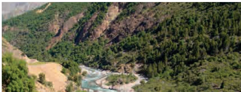
La Mina Run of the River Hydroelectric Project, VII Región
