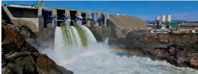
Angostura Reservoir Hydroelectric Project, VIII Región
