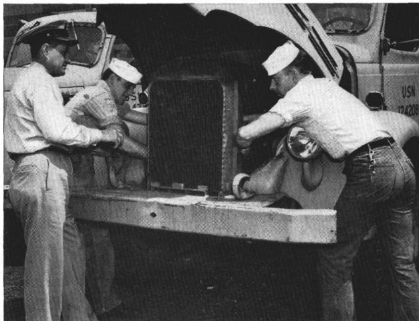
MOTORIZED equipment is kept in shapes by Seabee Reservists receiving truck maintenance training. They learn to service special equipment.
