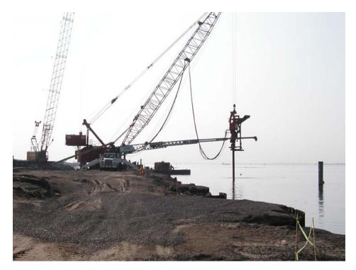
Photo 1: Installation of Stone Columns over Water
