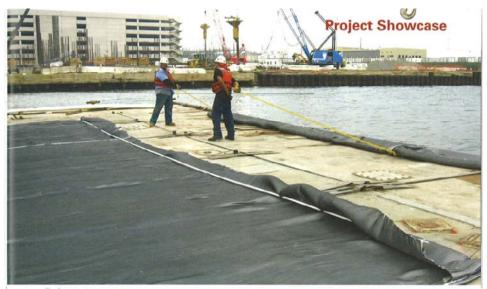
Photo 2: Deployment of Filter Fabric from Barge
