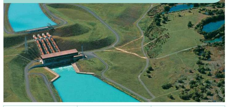
These 'twin' stations have the same generating capacity and similar equipment. Water from Lake Ruataniwha used by Ohau B goes into the Ohau C canal, which takes it to the Ohau C power station and out into Lake Benmore.
