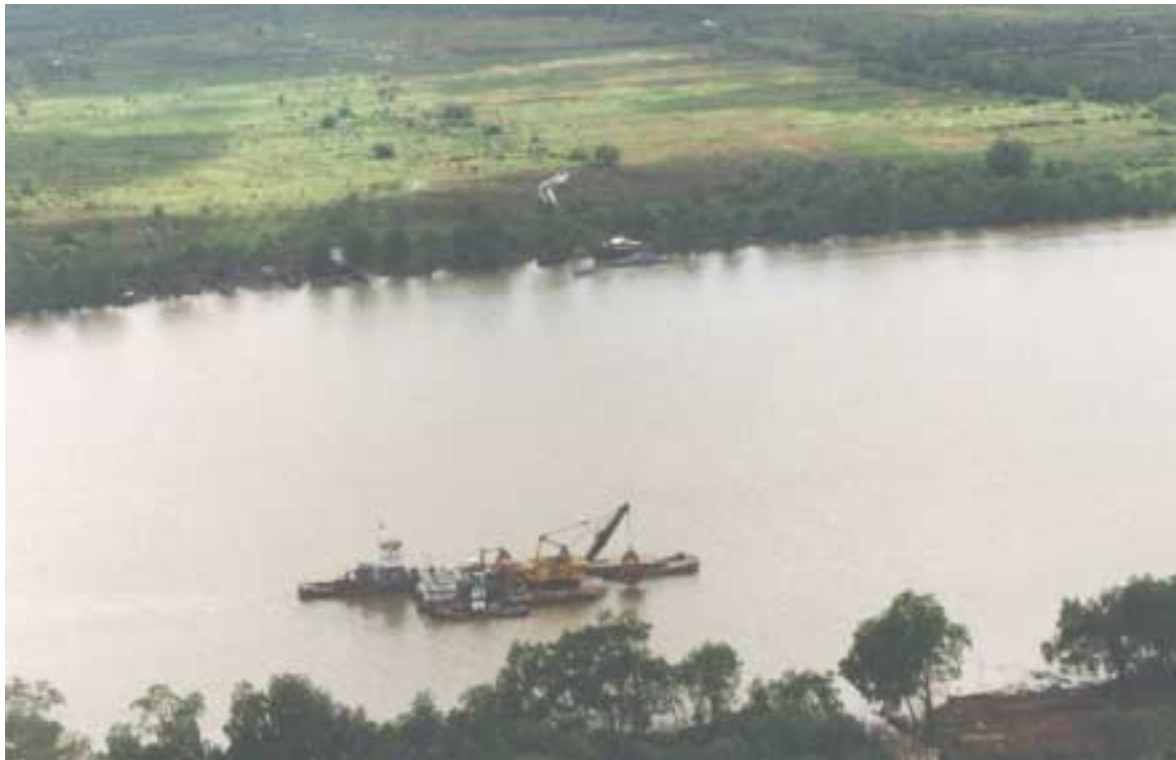
Figure 6.b Debris recovery using dredge
