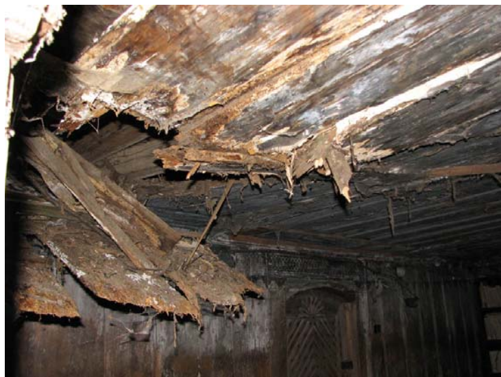
Figure 6 -Vault decayed by the Coniophora puteana and other fungi
