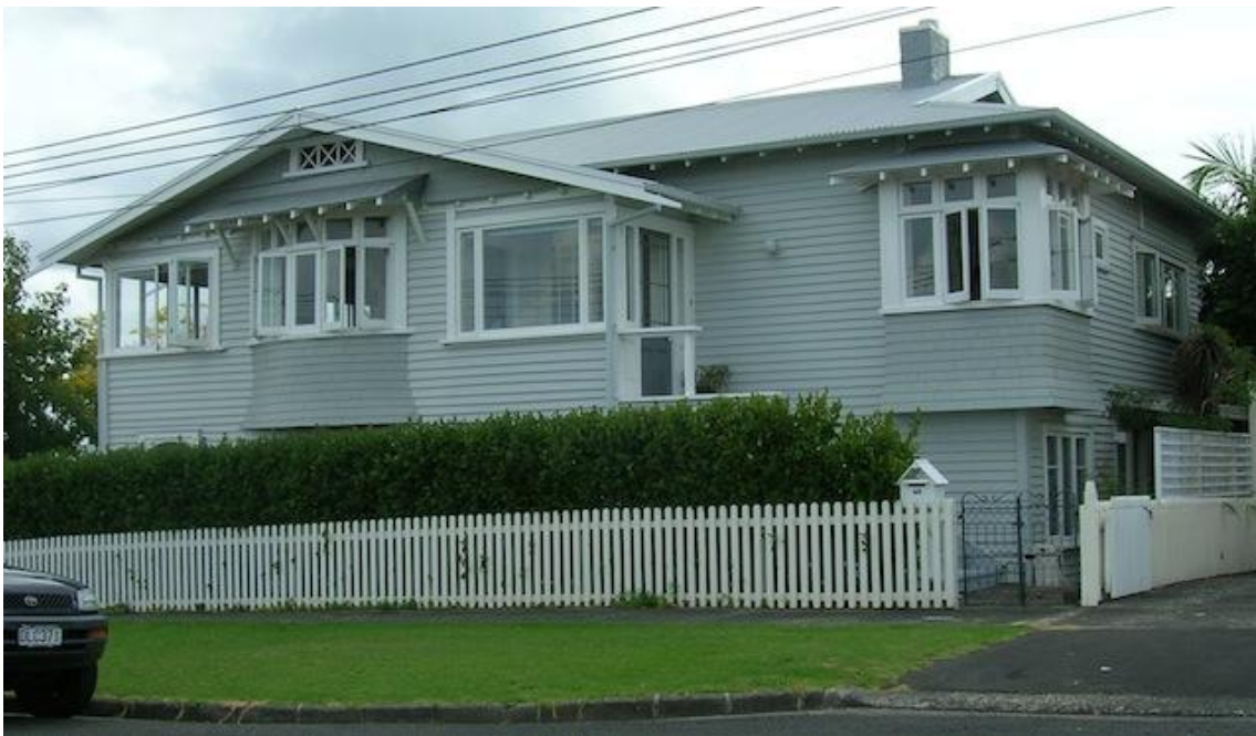
Fig. 20. Clarence Street bungalow, Salmond Reed Architects.
