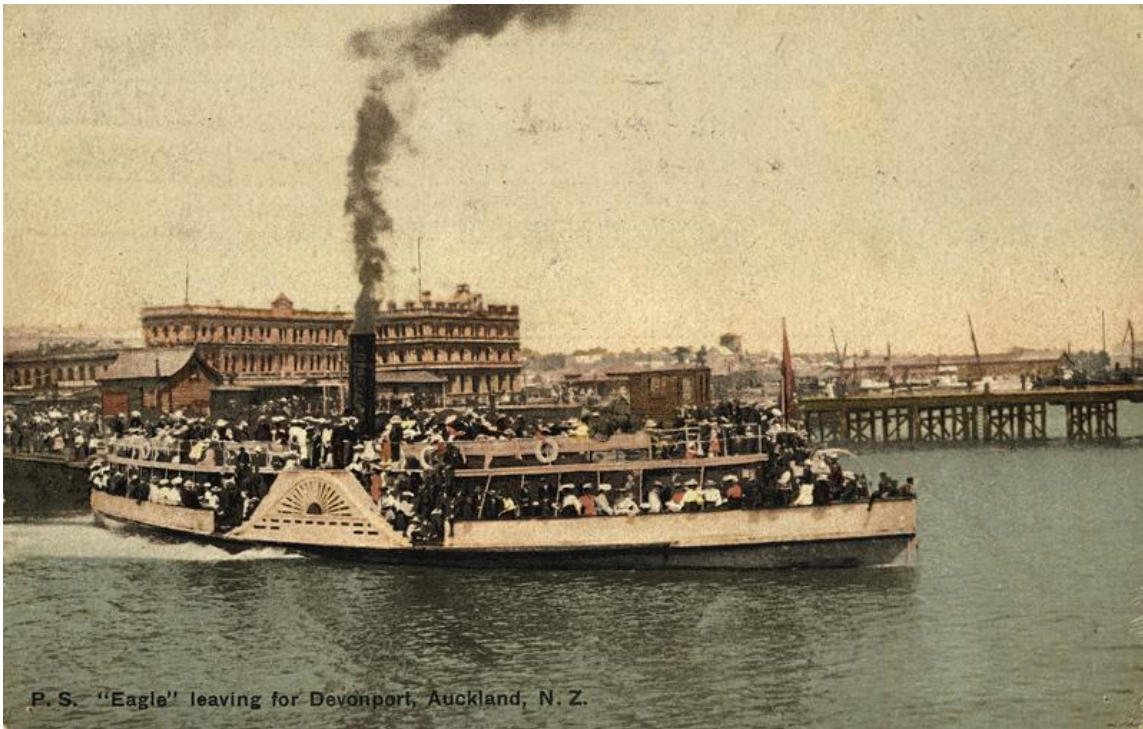
Fig. 4. PS Eagle leaving Auckland Wharf for Devonport, 1907. North Shore Libraries, NO110023.
