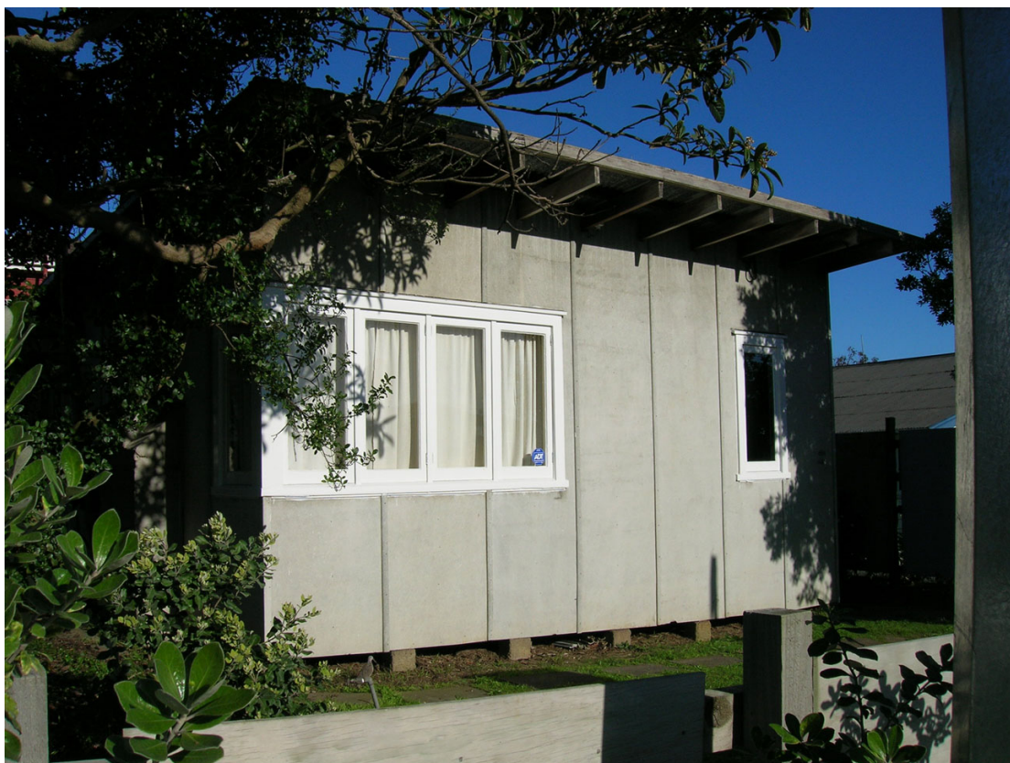
Fig. 36. Frank Sargeson's bach, Esmonde Road. Salmond Reed Architects.
