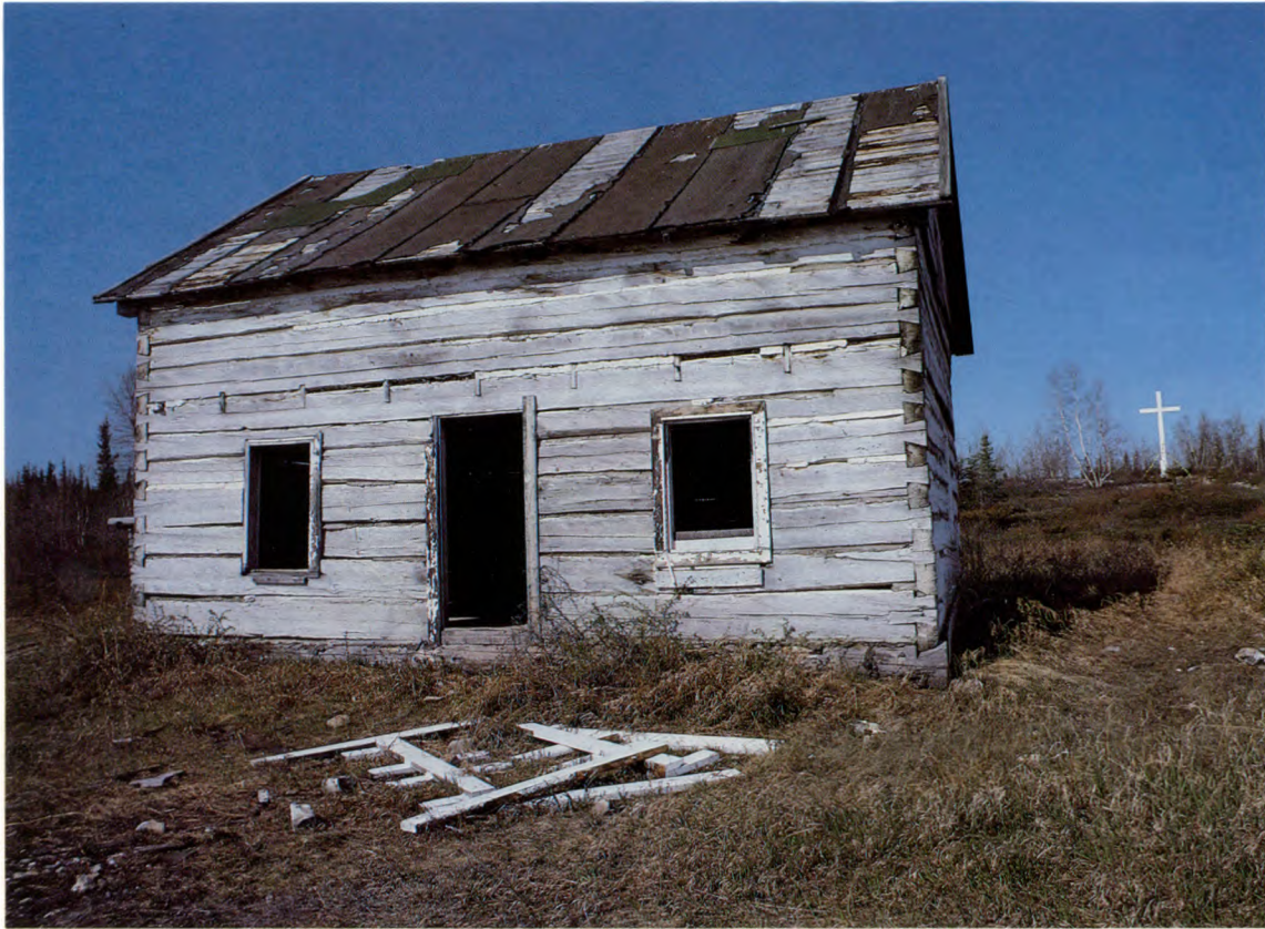
This building on Mission Island, near Fort Resolution, demonstrates building techniques still in use today.
