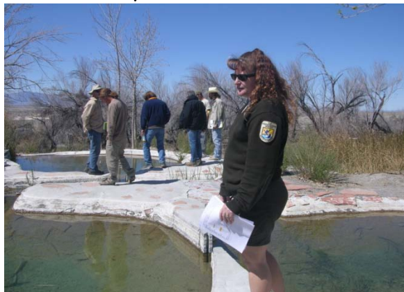
2006 - cement ponds at School Springs (built in early 80s)
