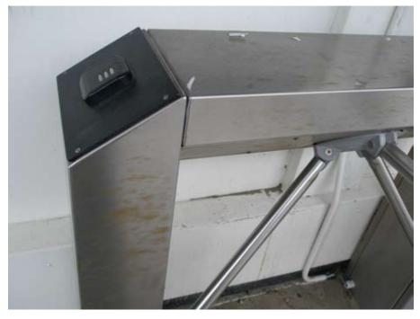
Fig. 2. RVS 316 access gate corroded by aerosols.
