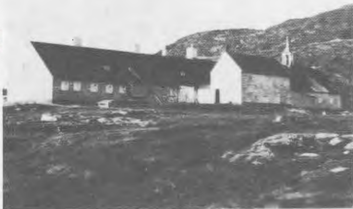
Abandoned Moravian buildings at Hebron
