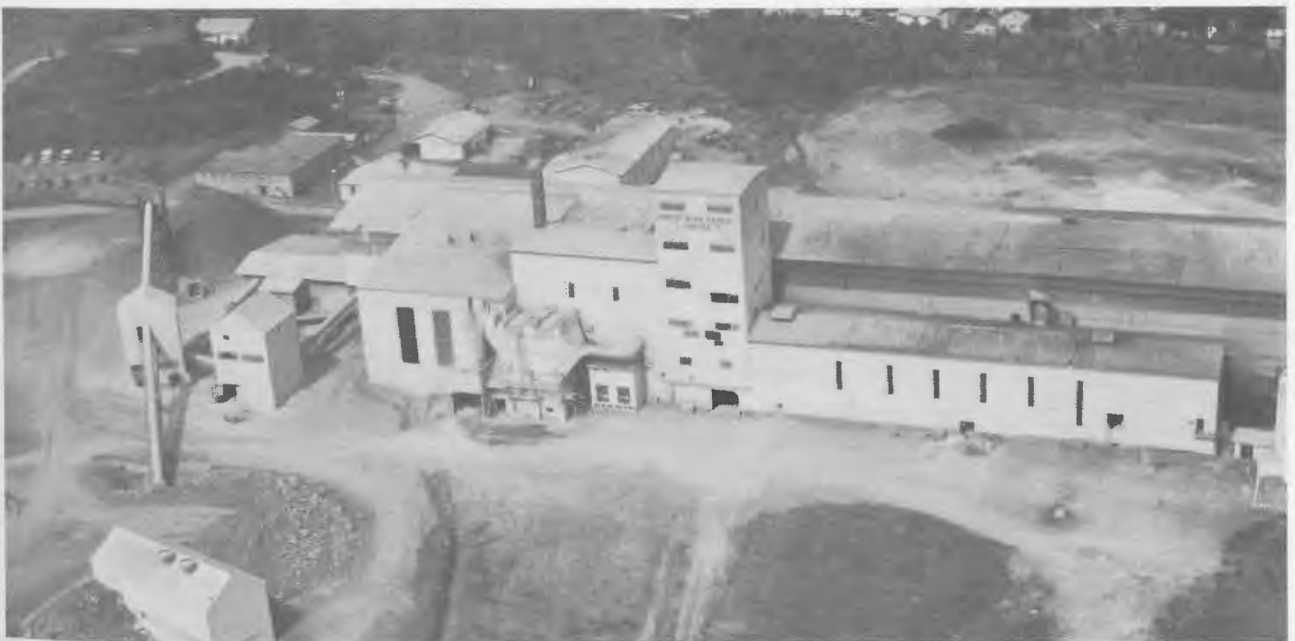
North Star Cement Ltd., Corner Brook
