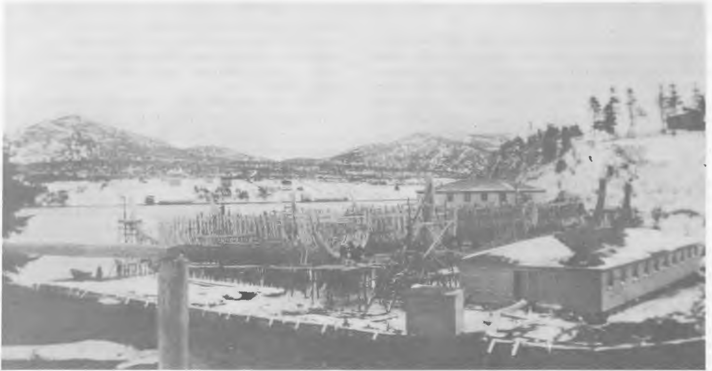
Schooner under construction at Marystown, 1939
