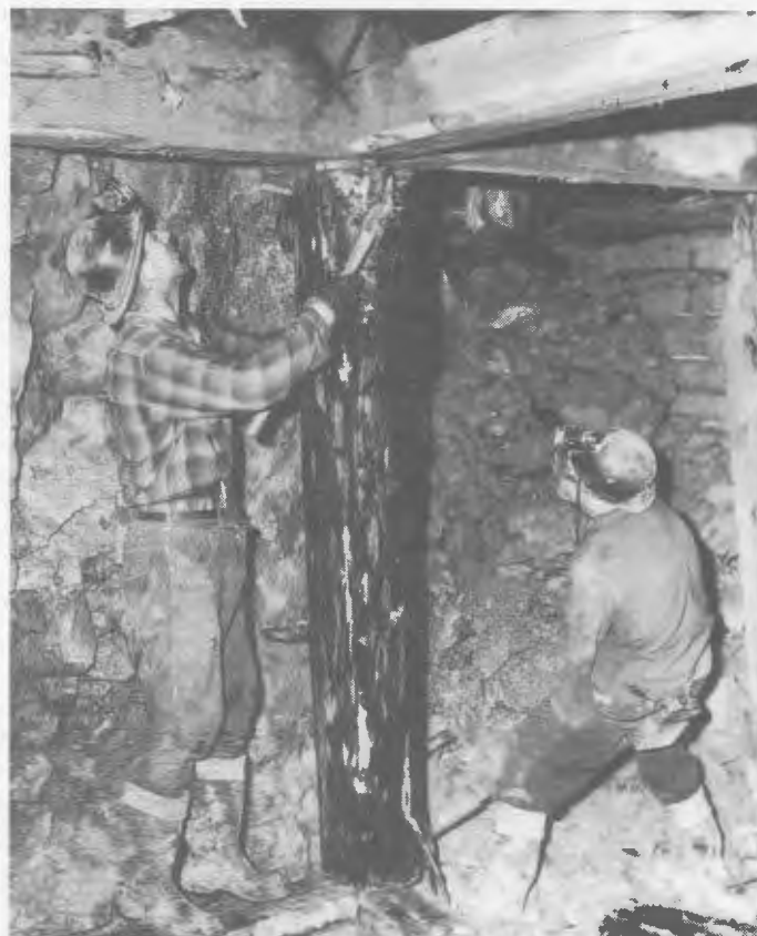
Timbering in Rothermere mine (Buchans)
