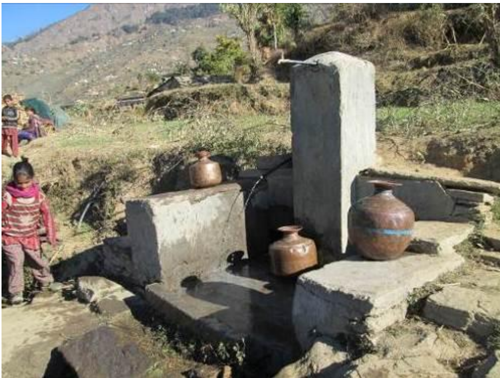
Tap stand at Kumalgaun W.S.P in KumalgaunVDC of Kalikot district
