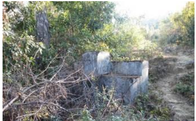
Non-functional tap stand in Katthur W.S.P. in Maohanyal VDC of Kailali
