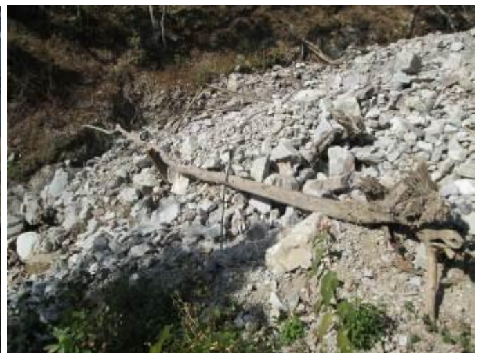
Pipeline disrupted by a landslide in Bajhadi W.S.P. in Hugsidir VDC of Baglung
