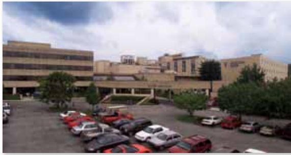
This aerial view shows the front entrance of the medical center prior to renovations.
