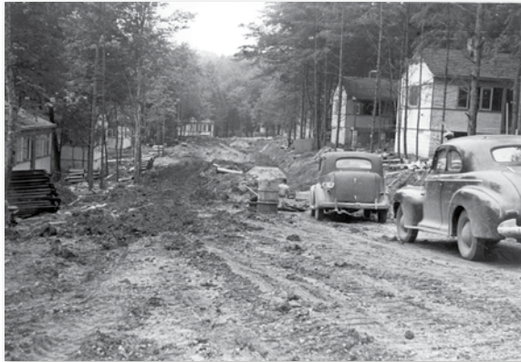
Construction and muddy streets made house calls difficult for Oak Ridge’s first physicians. This view of Tucker Road, looking east, shows the mud they had to contend with. Construction went on 24 hours a day. It wasn’t until 1946 that the town undertook a large-scale paving program. Photo by Ed Westcott
