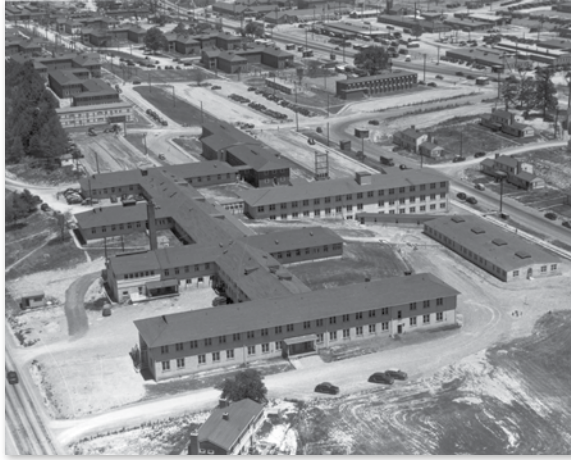
This aerial view of the first Oak Ridge Hospital looks east toward “Townsite.” The main entrance is at the front of the first wing. The second half-wing to the left is the Emergency Room, with its ambulance road down the hill to Tennessee Avenue, to the left. Nurses lived in Covington Hall, the white building at the upper left. Photo by Ed Westcott
