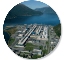
4 Hydro Aluminium Sunndal Primary aluminium Capacity: 390 000 tons
