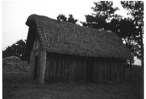
Fig 1. Reconstruction of a typical wooden framed early Anglo-Saxon house at West Stow, Suffolk.
