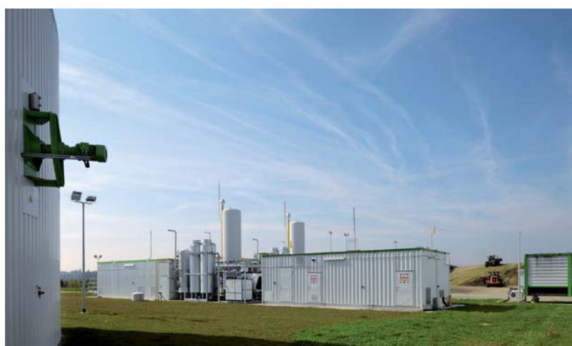
Upgrading plant for biomethane, space-efficient installation in standard containers
