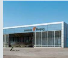
Ameco A380 Hangar Beijing, China
