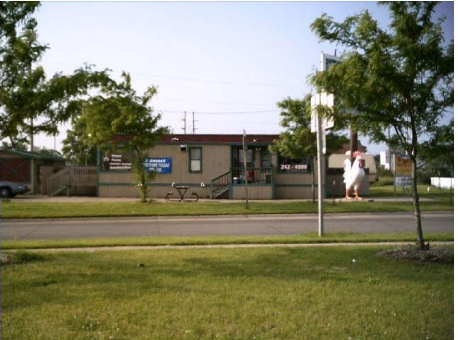
City of Clinton, 1101 - 1105 South 4th St.
