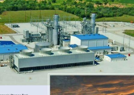
the combustion turbine heating water to make steam to power the steam turbine), and the combined efficiency becomes 58 percent.
