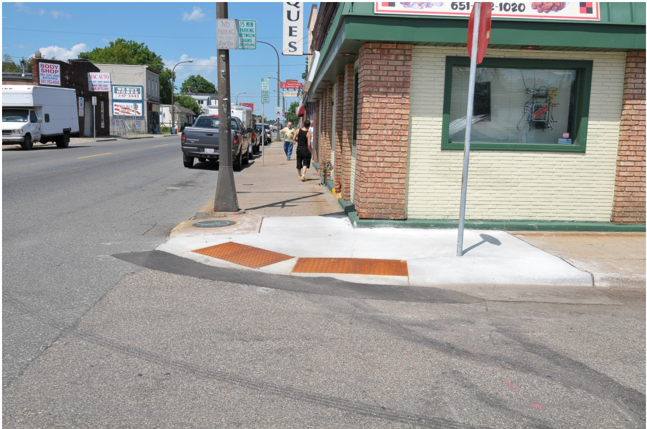
ADA compliant curb cut
