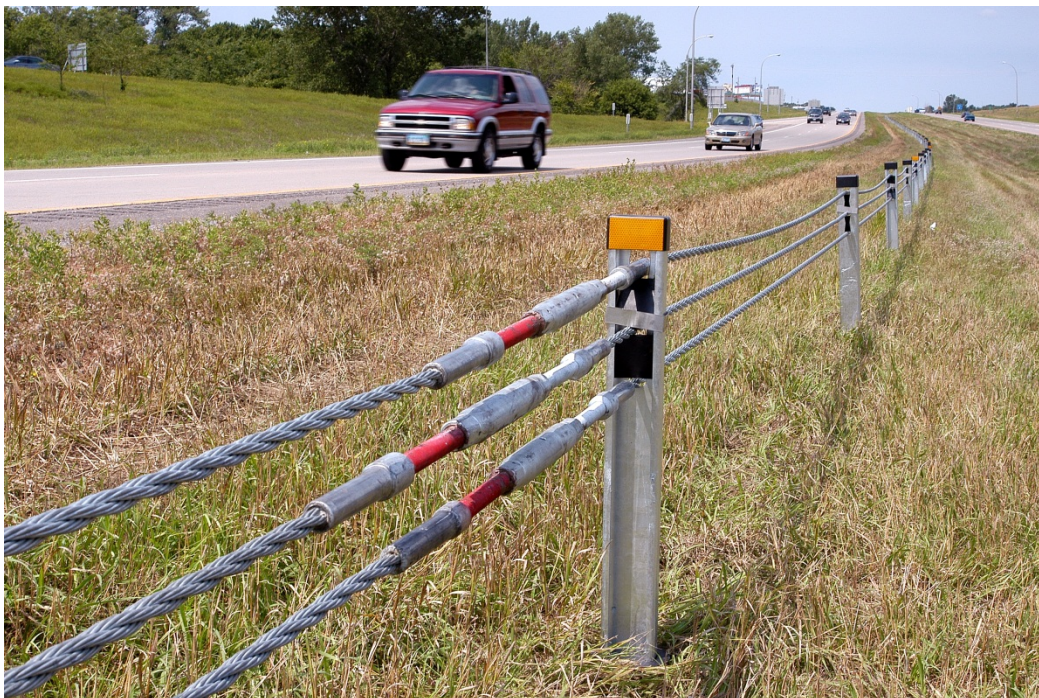
Cable median barrier
