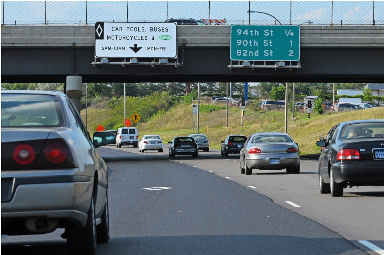
High occupancy vehicle lane
