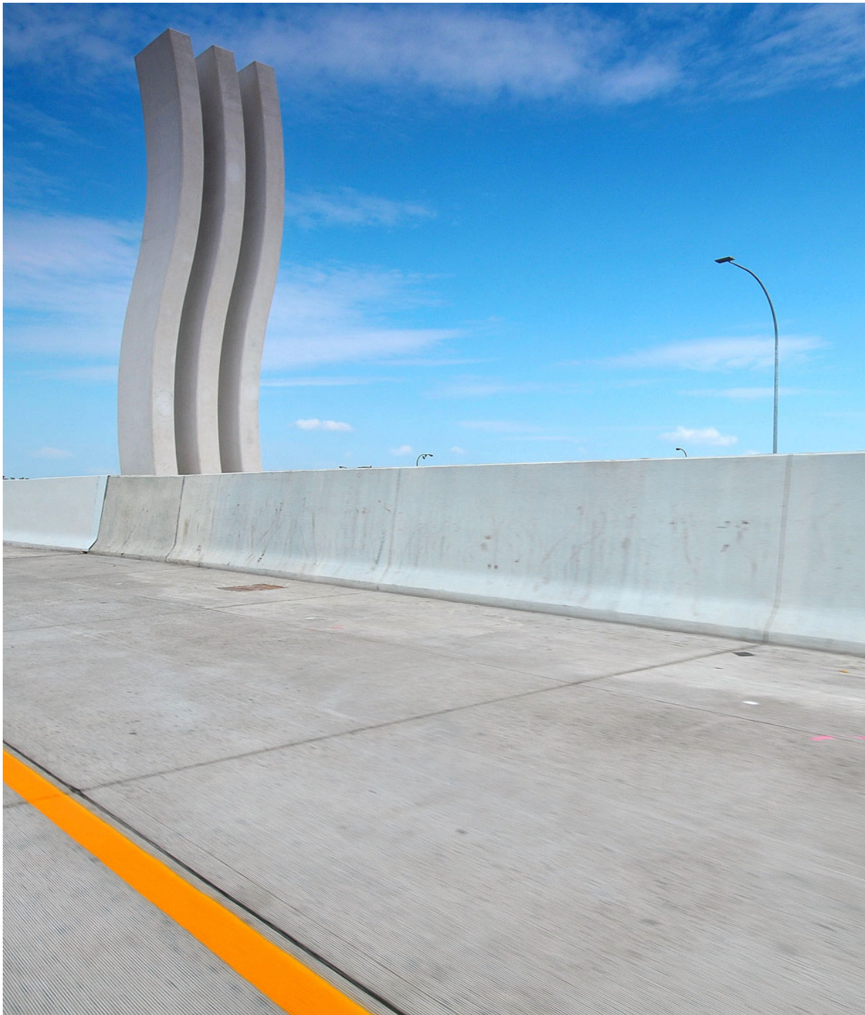
Roadway with tall concrete median barrier
