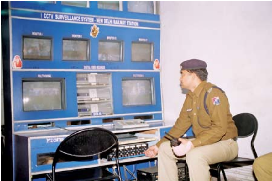
CCTV surveillance system, New Delhi Railway Station, Northern Railway.
