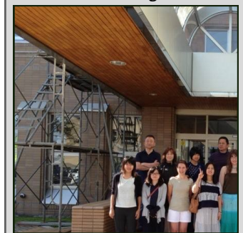
Scaffolding at City Hall
