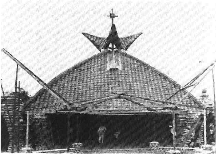
Fig. 9a: Pohsarang Catholic Church, Kediri. Front elevation as photographed in the 1930s
