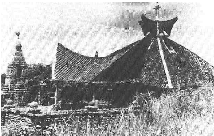
Fig. 9b: Pohsarang Catholic Church, Kediri. Side elevation as photographed in the 1930s
