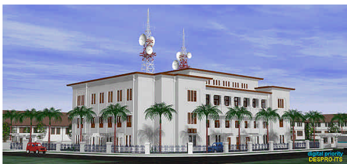
Fig. 5b: Telecommunication Office, Surabaya
