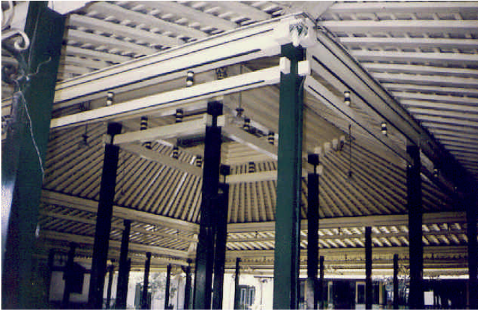
Fig. 8a: Javanese construction as shown in the Open Pavillion, Yogyakarta Palace. Note that for both for Fig 8a and 8b, the outward appearance of the roof form is quite similar to Fig 3.
