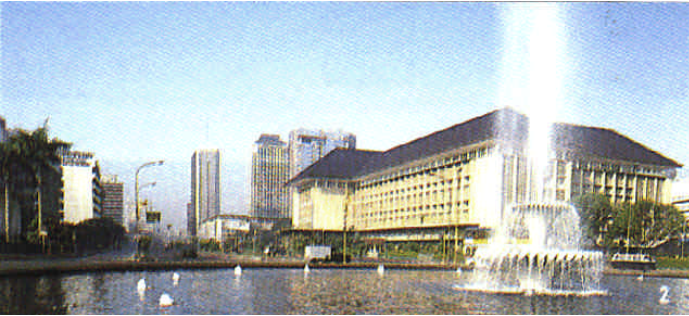
Fig. 10: Bank Indonesia Building, Jakarta
