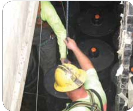
Replacing stormwater filters
