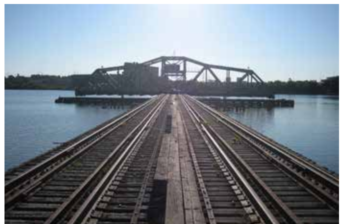
Historic CSX bridge
