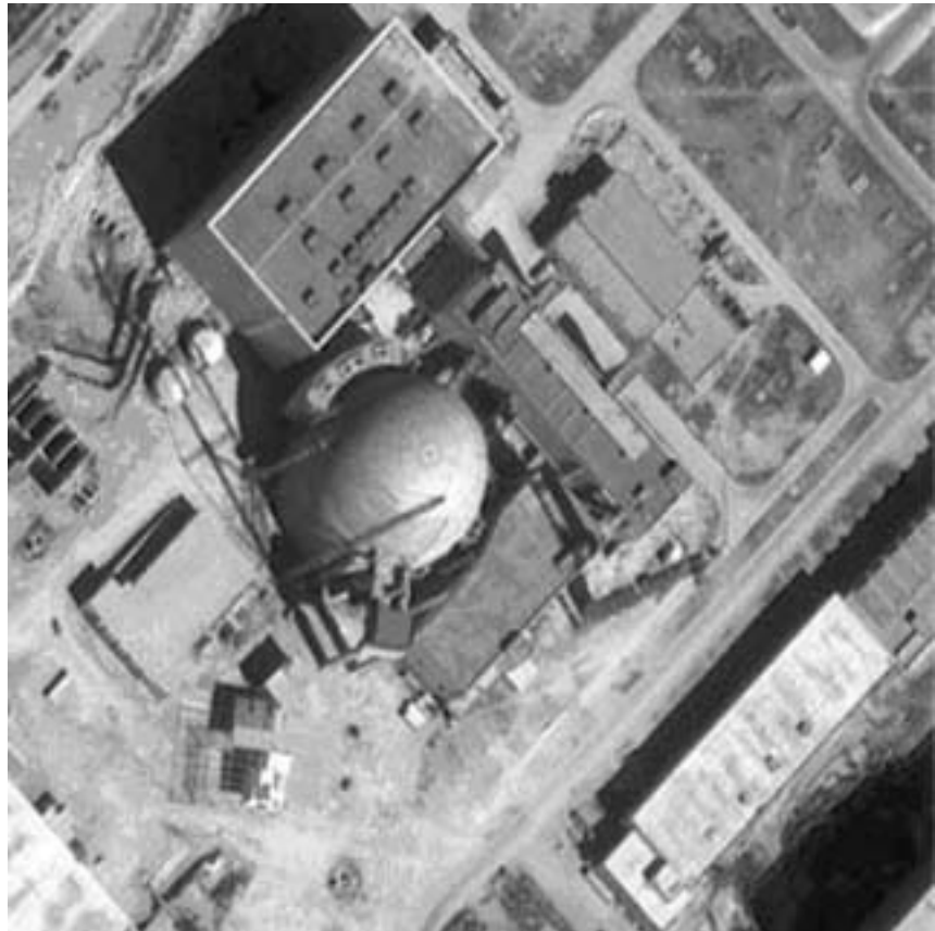
Bushehr Reactor in Iran.
