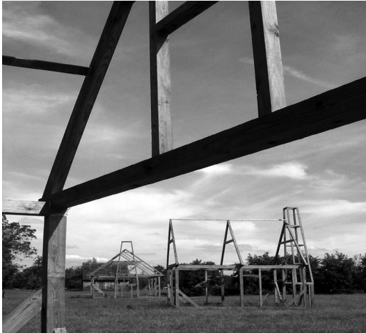
“Ghost” frames erected in 1994 mark the location of actual colonial buildings. (Courtesy Historic St. Mary’s City)
