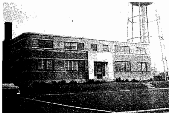
Office Building looking North
