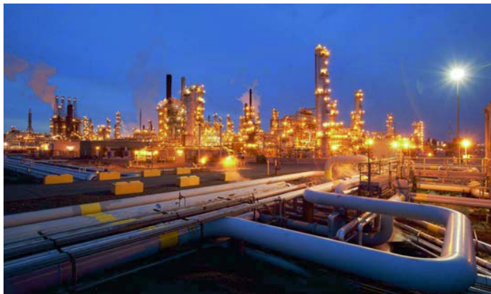
▲ Cherry Point refinery processes around 230,000 barrels of crude oil per day, primarily for transportation fuels.
