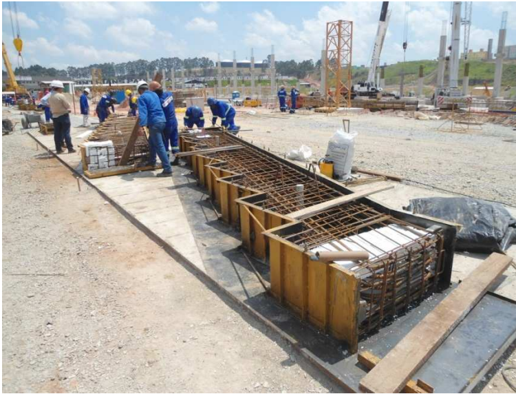
Figure 5. Assembly of precast grandstands prefabricated beams on site.
