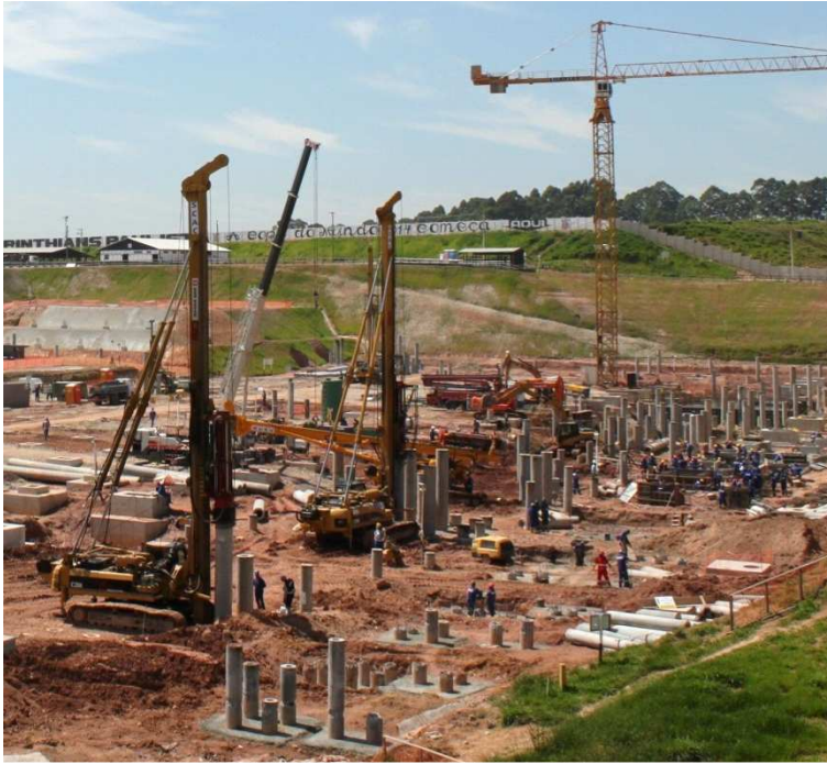
Figure 7. Pile driving
