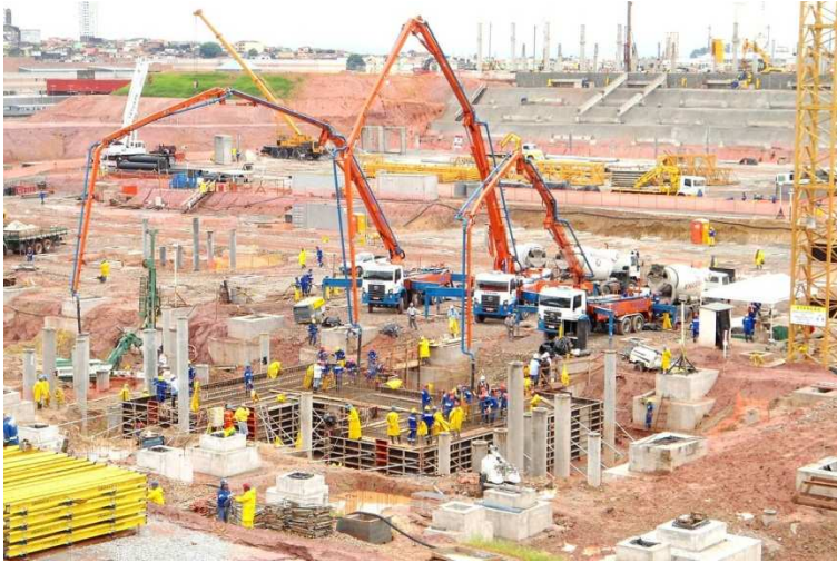
Figure 9. The cap piles were cast in situ.
