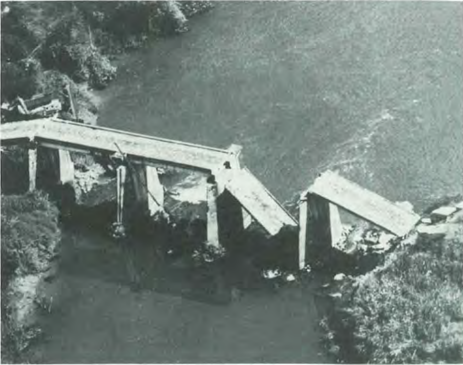
A Destroyed Bridge in Laos, 1965
