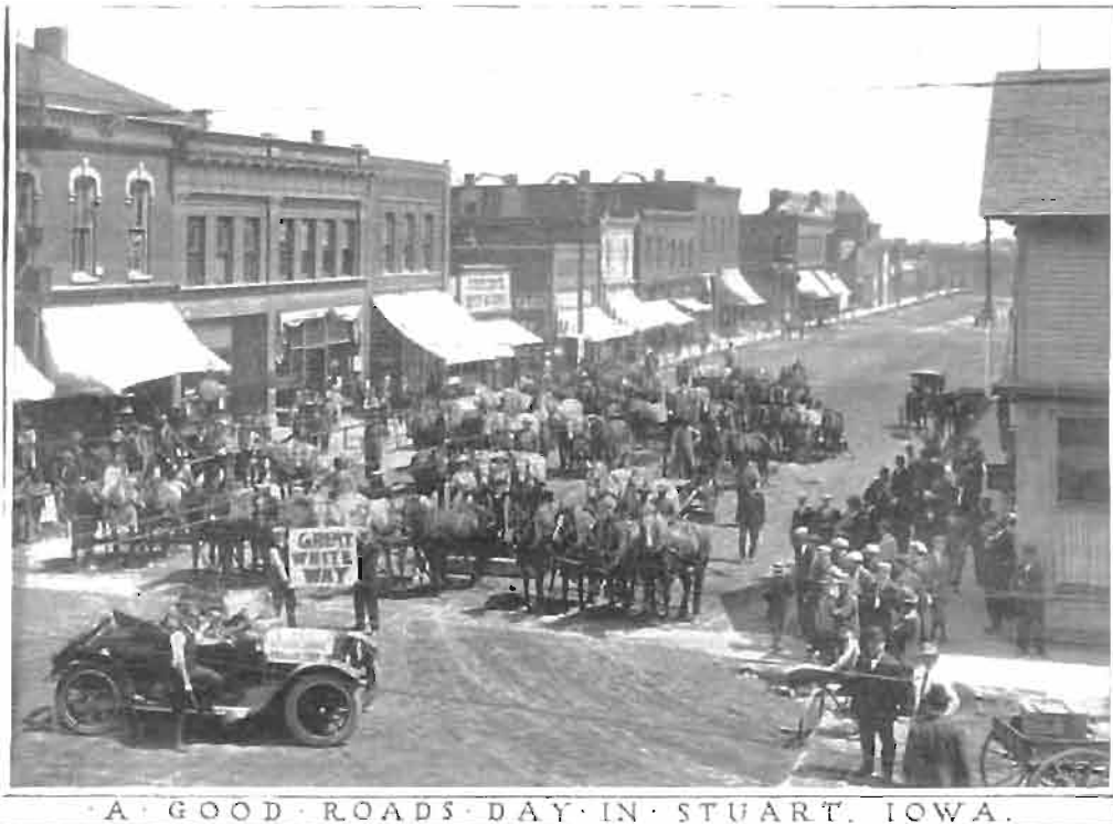
Undated photograph road dragging activity along Nassau St. (now 2 nd ), Stuart's historic main street shopping district located one block north of the Sexton Hotel. This view looks east. (Iowa Department of Transportation. Accessed at http://historicalphotos.iowadot.gov/ )
